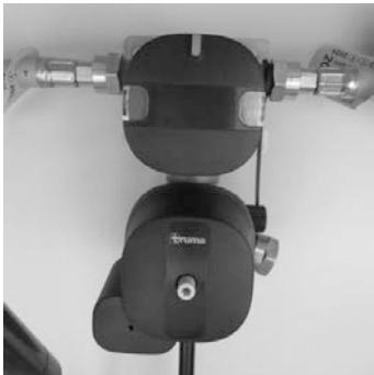
Fig. 74: Gas supply (with Eis-Ex and remote control)
